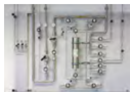
Gas bottle and distribution Cabinets
