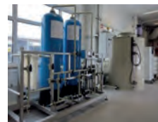
Chemical distribution DI Water system
