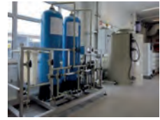
Chemical distribution DI Water system
