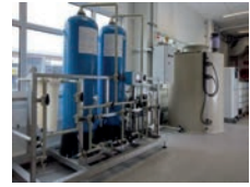
Chemical distribution DI Water system
