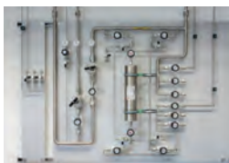
Gas bottle and distribution Cabinets
