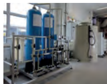
Chemical distribution DI Water system
