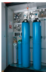
Gas bottle and distribution Cabinets
